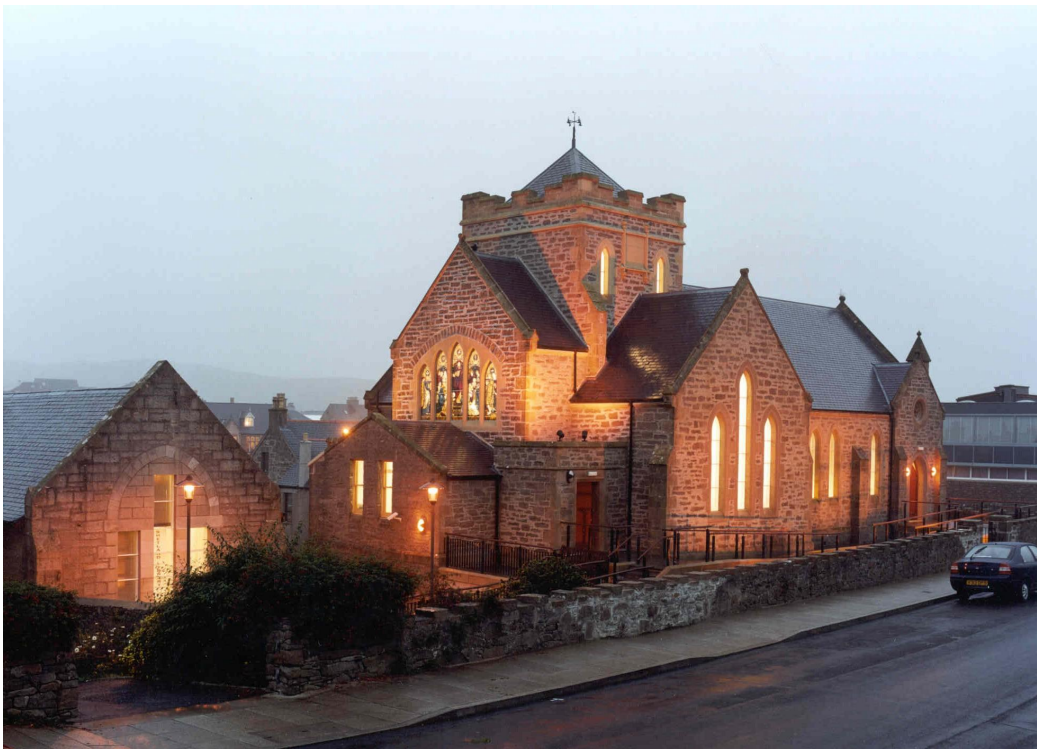
New Shetland Library and Learning Centre floodlit in early evening.
